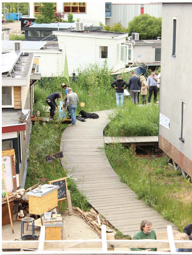
Fig. 1. For a 10 year period completely renovated and insulated houseboats have been installed for use as offices for a group of creative initiators at De Ceuvel in Amsterdam, The Netherlands
